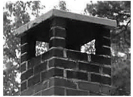
Concrete Cap Chimney Top
